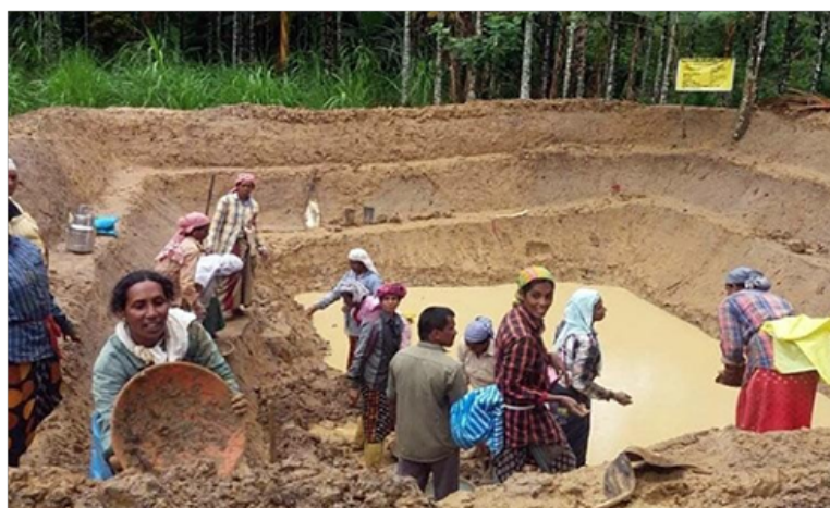
Pond construction, Kaniyambetta GP, Wayanad by MGNREGA workers.
